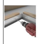
Secure the ceiling frame to ceiling by driving screws through ceiling frame collar into joists/ trusses if available.
